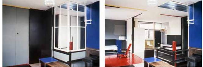
Fig. 1. An example of reconfigurable rooms from early 20th-century architecture: two physical configurations, same view, of the Rietveld House (1924, Utrecht) showing manually movable shutters and panels dividing the space (left) and, retracted (right), opening-up the space.
